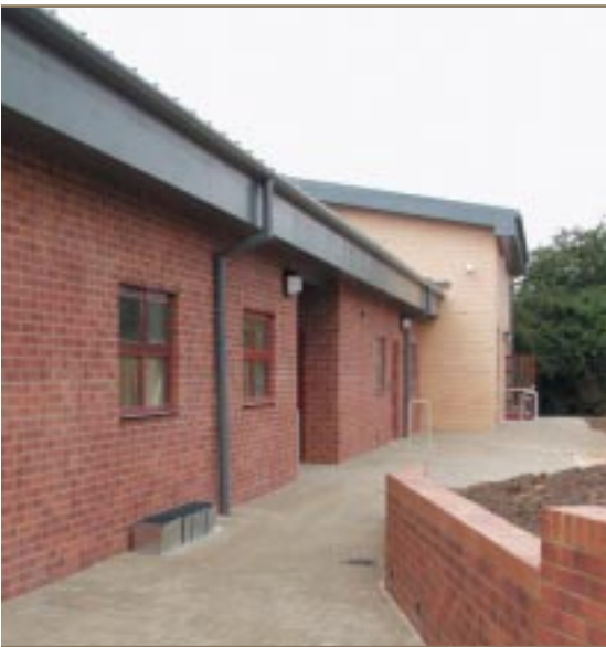
CONSTRUCTION NEARS COMPLETION ON THE NEW SCHOOL
