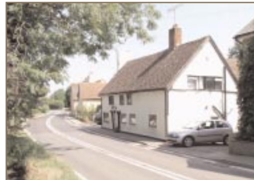
ABOVE: DASSELS LOOKING NORTH
