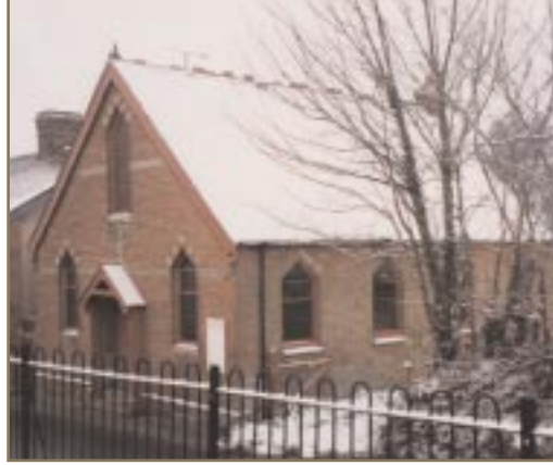
LEFT: BRAUGHING METHODIST CHURCH
